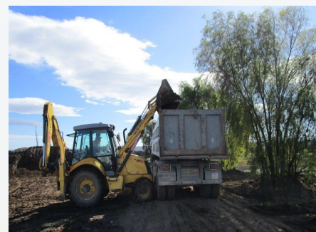
Loading mud from a recycling plant
